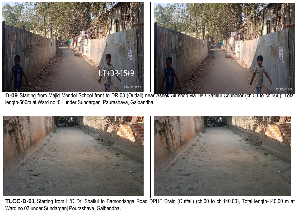
Figure 3:Existing Roads and Drains Picture
